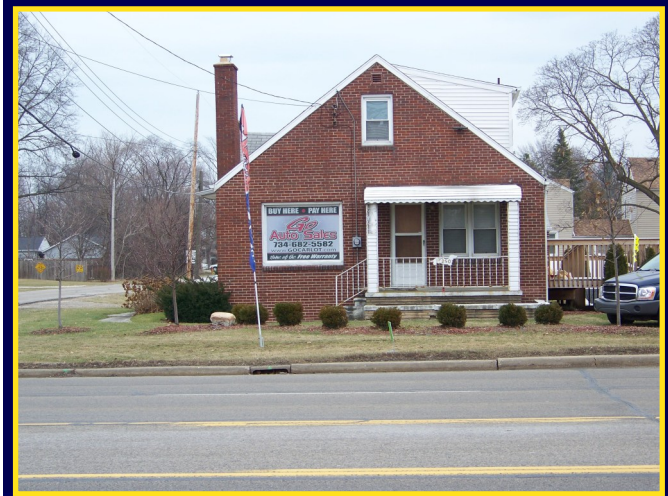
WEST ELEVATION OF MAIN BUILDING
