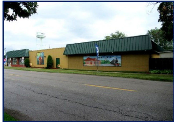
VIEW OF BUILDING FROM MAIN STREET LOOKING SOUTHEAST
