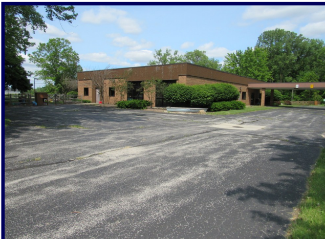
WEST FAÇADE & SOUTH CANOPY ENTRANCE/EXIT
