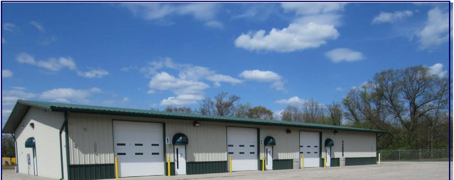
FRONT FACADE (SOUTH) WITH THREE OVERHEAD DOORS AND THREE MAN DOORS
