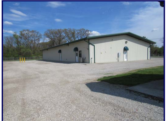
WEST AND NORTH FACADE
