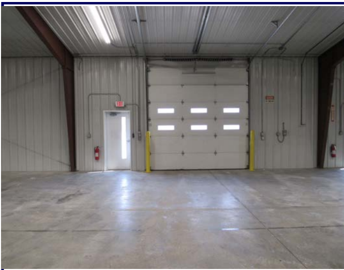
SOUTH (FRONT) 12' OVERHEAD DOOR
