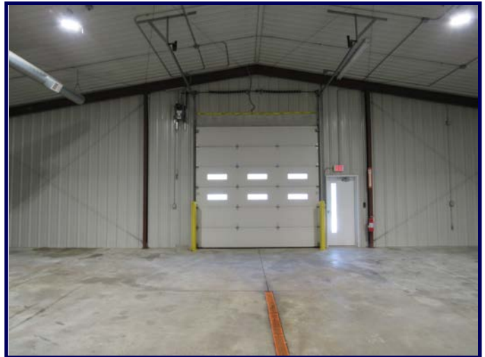
EAST 12' OVERHEAD DOOR
